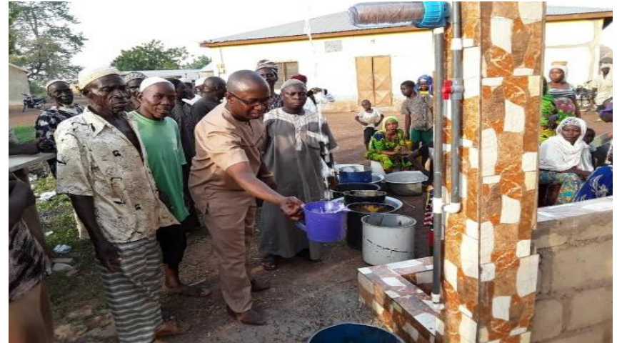
Mechanized Borehole and Extension of Stand Pipe Water facilities to Kigbiripe
