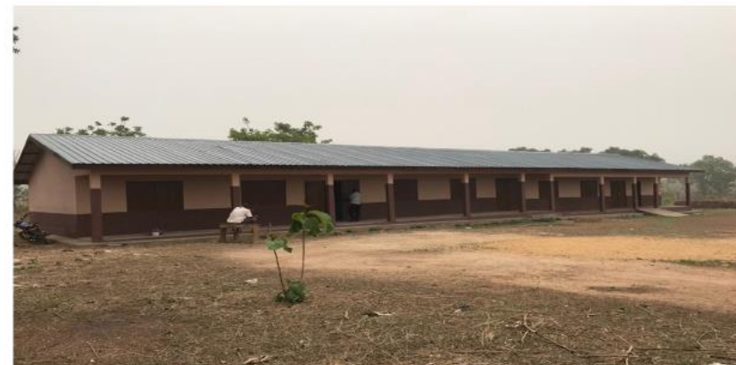
1NO. 3UNIT CLASSROOM BLOCK COMPLETED AT GBORSIKE
