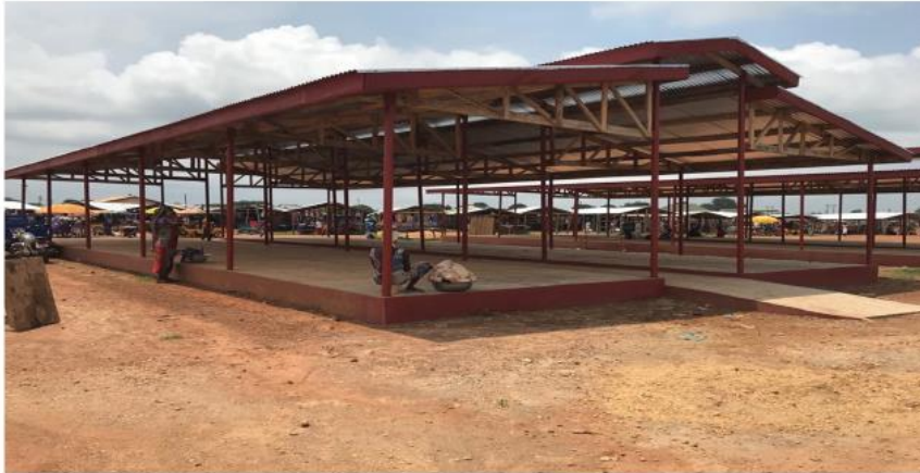
2NO. 40UNIT MARKET SHEDS COMPLETED AT KPASA NEW MARKET
