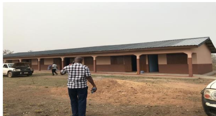
1NO. 3UNIT CLASSROOM BLOCK COMPLETED AT NANJINGON
