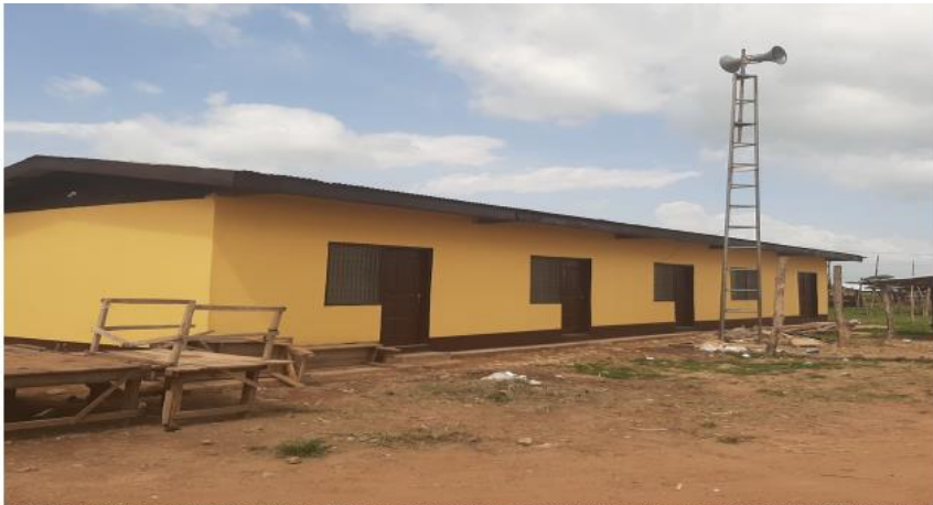
REVENUE AND INFORMATION CENTRE REHABILITATED AT KPASSA NEW MARKET
