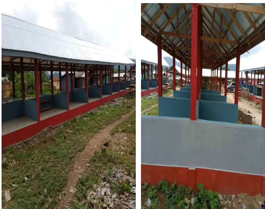
Rehabilitated 3No. Market Stalls at Papase Market
