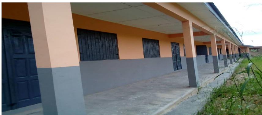
Constructed 3-unit classroom block at KASEC JHS (Kadjebi)
