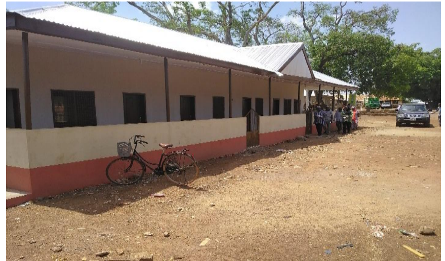
Rehabilitation of Environmental Health and sanitation Unit Office in Yendi
