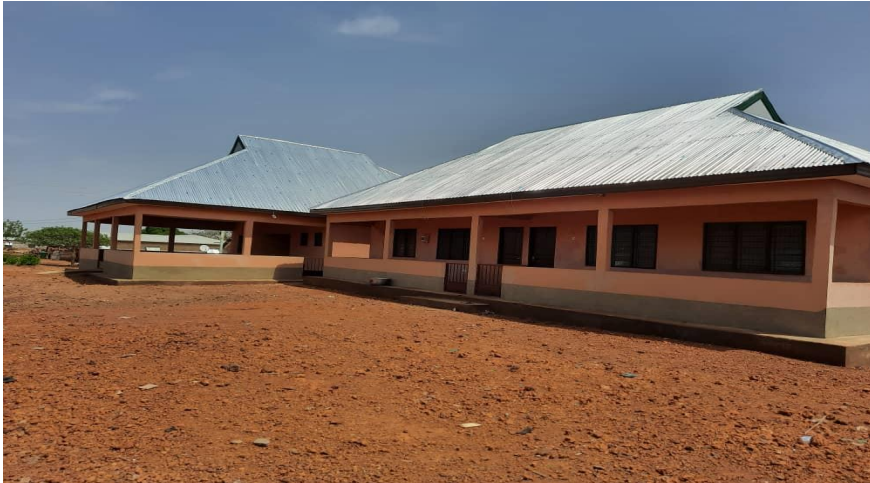
Constructed 1no. CHPS Compound at Wali Yapala
