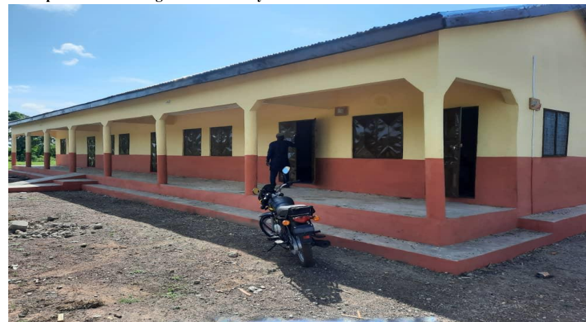
Constructed and Furnished 3-Unit classroom block, with office, store, 4- seater KVIP and 2-unit open urinal at Yingsala community
