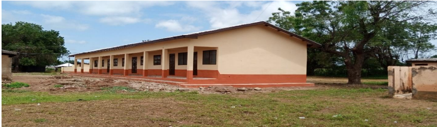
Figure 1. Construction of 1 No. 3 Unit Classroom block with ancillary facilities at Diare
