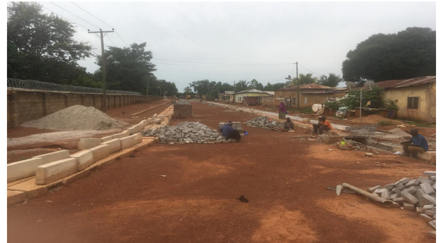
Above: Construction of 0.75Km road at Ward-K
