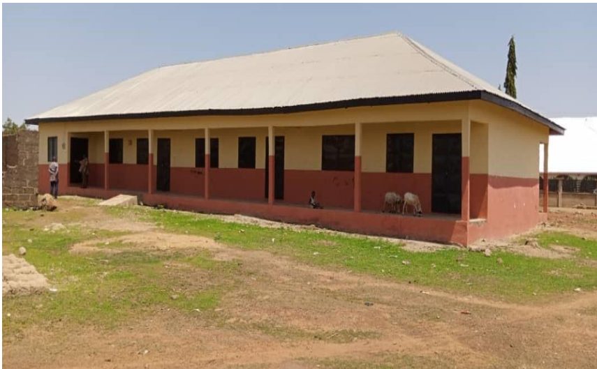
Above: 3- Unit Classroom Block at Failatu JHS.
