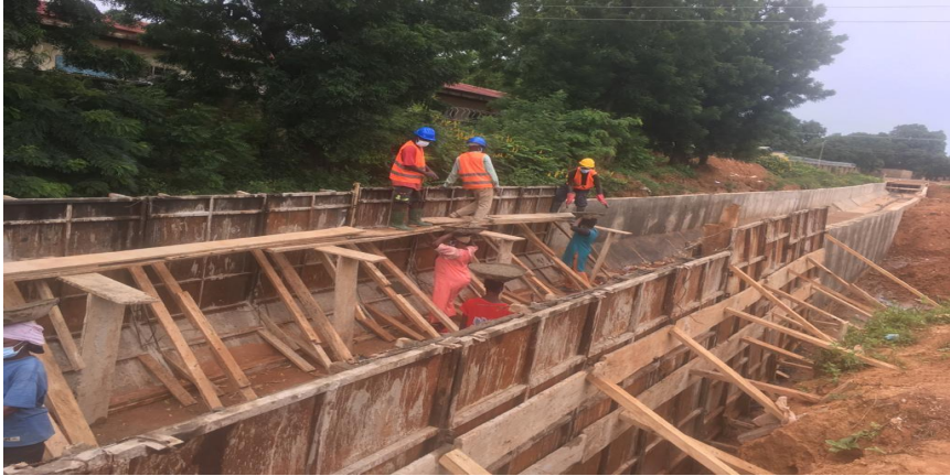
Above & Below: Construction of Storm Drains at Ward-K.
