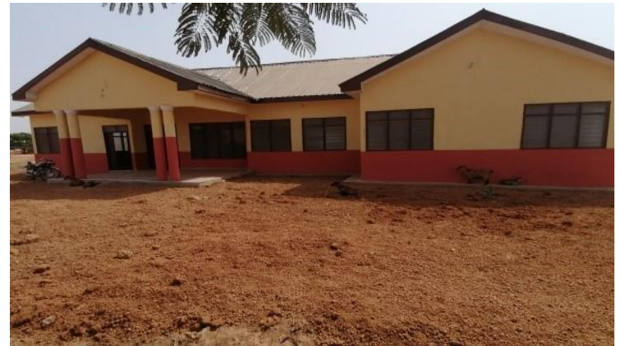
Above: Construction of Clinic at Shishegu.
