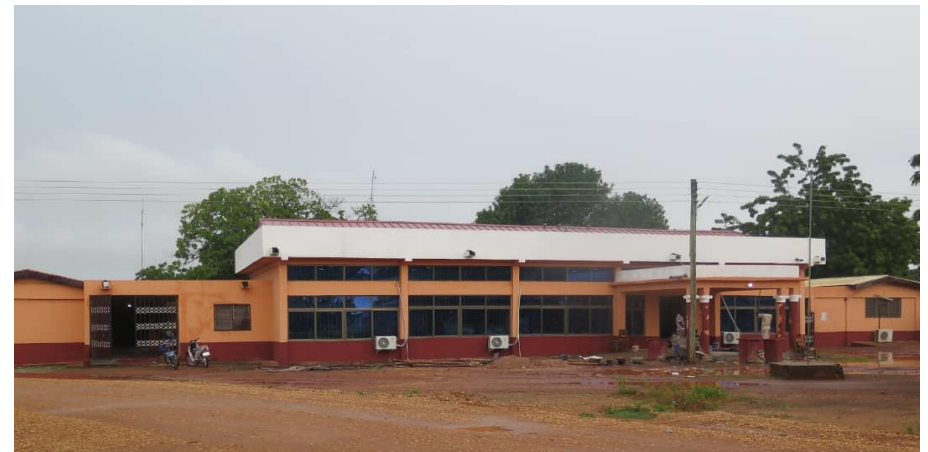
Renovated Saboba District Assembly Hall
