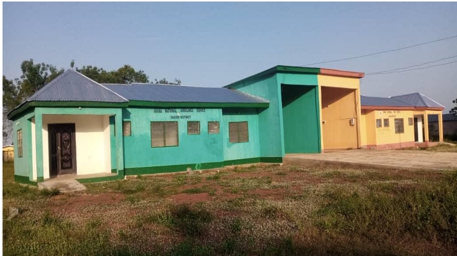
Newly Constructed Fire and Ambulance Stations
