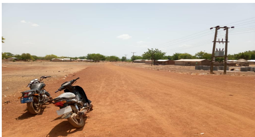
Rehabilitated Kpatinga – Bugnayili Feeder road
