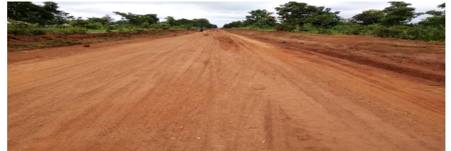
Reshaped Nasande-Wanbondam- Tindang feeder road
