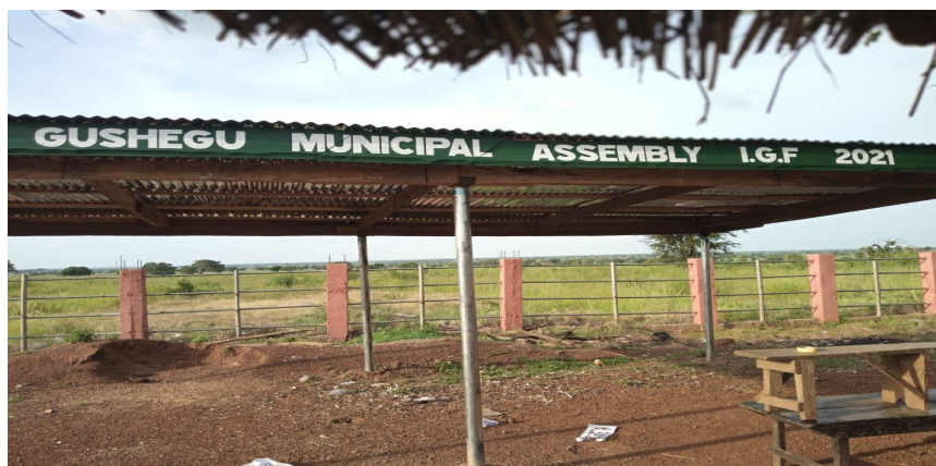
Constructed 2n0.6unit Open shed at Gushegu Cattle Market
