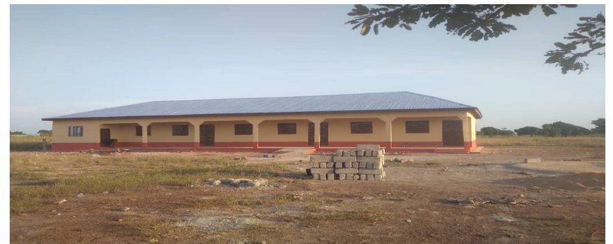
Completed Construction of 1no.3unit Classroom Block at Kpisinga
