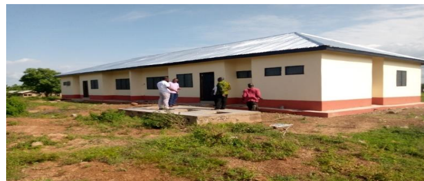
Constructed 2no.semi – detached bungalow at Gushegu
