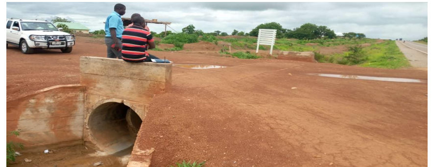
Completed Construction of 1200mm access pipe culvert to Gushegu cattle market
