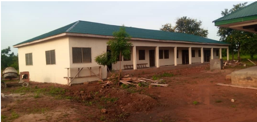
Construction and Furnishing of 3unit classroom block at Langbinsi
