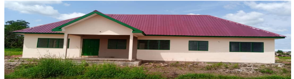
Completed Teachers Quarters at Gambaga
