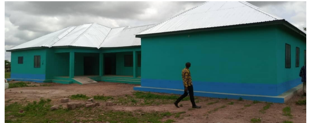
Completed CHPS Compound at Yankazia
