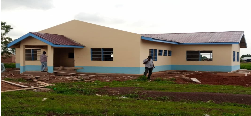
Construction of Maternity Block at Langbinsi
