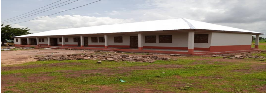
Completed and furnished 3unit classroom block at Sakogu
