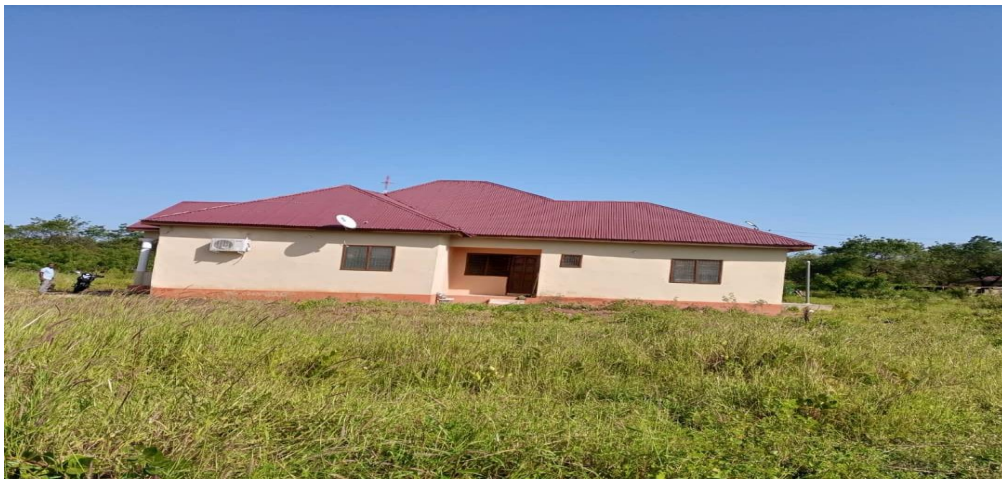
Completed and Furnished Doctor Bungalow at Gambaga
