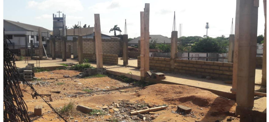
Construction of 6-unit classroom block at Tesano
