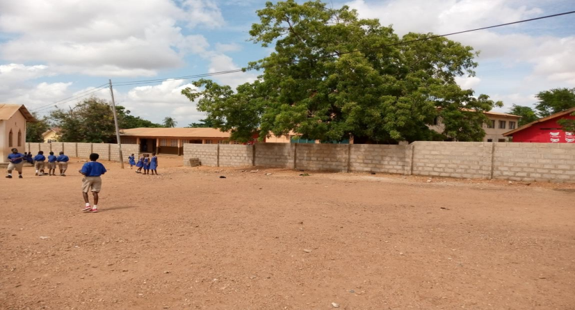
CONSTRUCTION OF DIVISIONAL FENCE WALL AROUND THE ASHONGMAN PRESBYTERIAN BASIC SCHOOL
