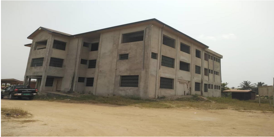
F.2 CONSTRUCTION OF HOSPITAL AT ABLEKUMA ABEASE
