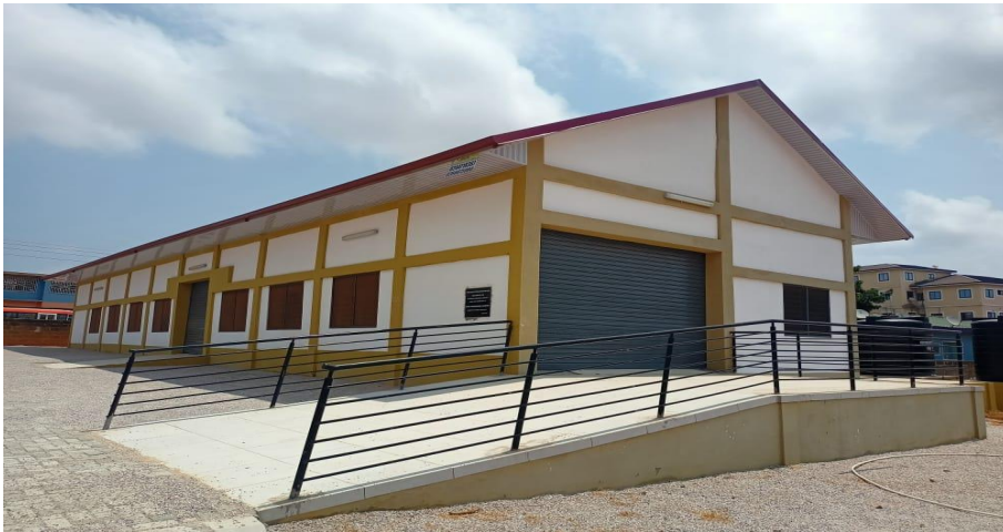
F.3 CONSTRUCTION OF BOTTLED & SACHET WATER FACTORY AT ANYAA.
