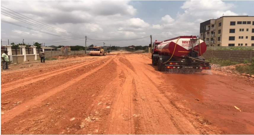
REHABILITATED COMMANDOS AND MAMOMO AREA ROADS- ADENTAN (2.00 KM)
