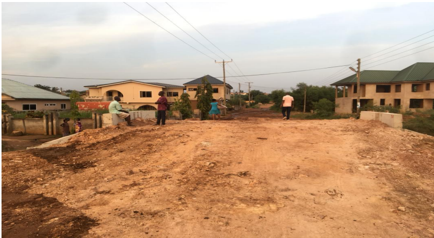
CONSTRUCTED 2X2 BOX CULVERT AT FAFRAHA
