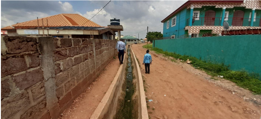
CONSTRUCTED U-DRAIN AT NEW LEGON
