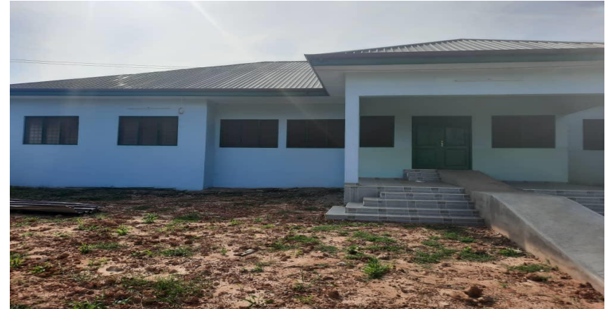
CONSTRUCTED 1 NO. MATERNITY BLOCK AT FAFRAHA
