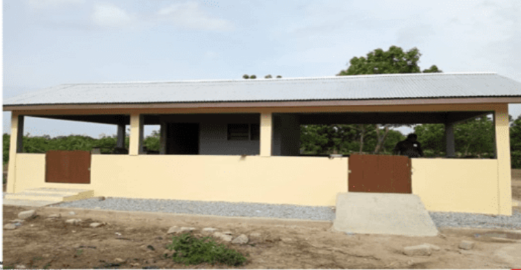
CONSTRUCTED SCHOOL FEEDING KITCHEN AT CESARKOPE (DACF-RFG, 100%)
