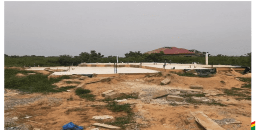
20% DCE'S BUNGALOW STILL UNDER CONSTRUCTION (DACF)
