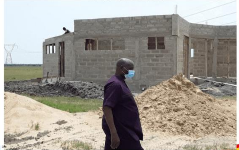
60% CONSTRUCTION OF 1 NO. MODERN SLAUGHTER HOUSE (DACF-RFG)
