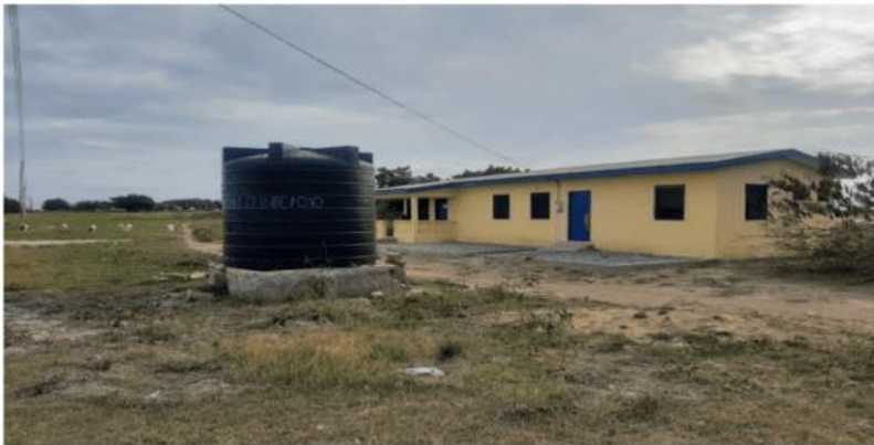
RENOVATED CHPS COMPOUND AT MADAVUNU (DACF, 100%)
