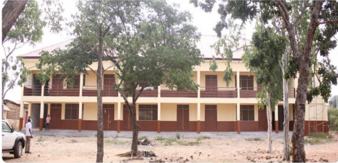
CONSTRUCTION OF 1 NO. 2 STOREY 6 UNIT CLASSROOM BLOCK AT SOMANYA METHODIST – DACF RGF - 100% COMPLETED
