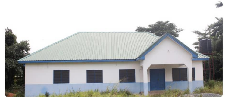
CONSTRUCTION OF 1 NO. CHPS COMPOUND AT AKORWU BARNA - DACF (100% COMPLETED)
