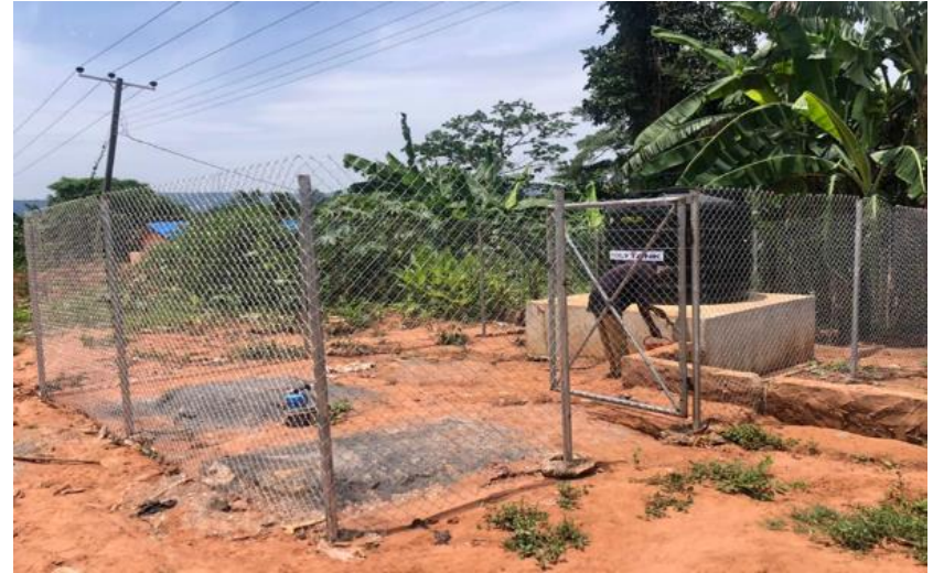
Borehole at Asaasekokor
