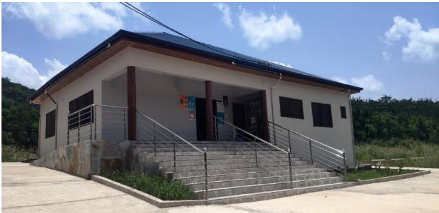
CHPS Centre constructed at Abonse
