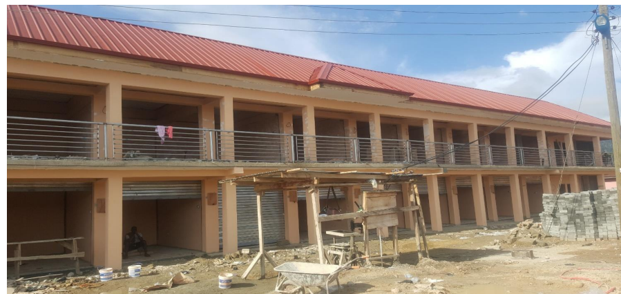
Picture 1: 44 No. 2 storey lockable stores at Nkawkaw Adom Market
