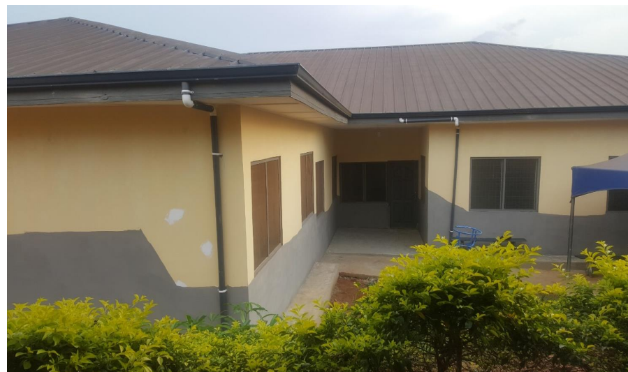
Picture 2: Newly constructed Nkawkaw Health Centre
