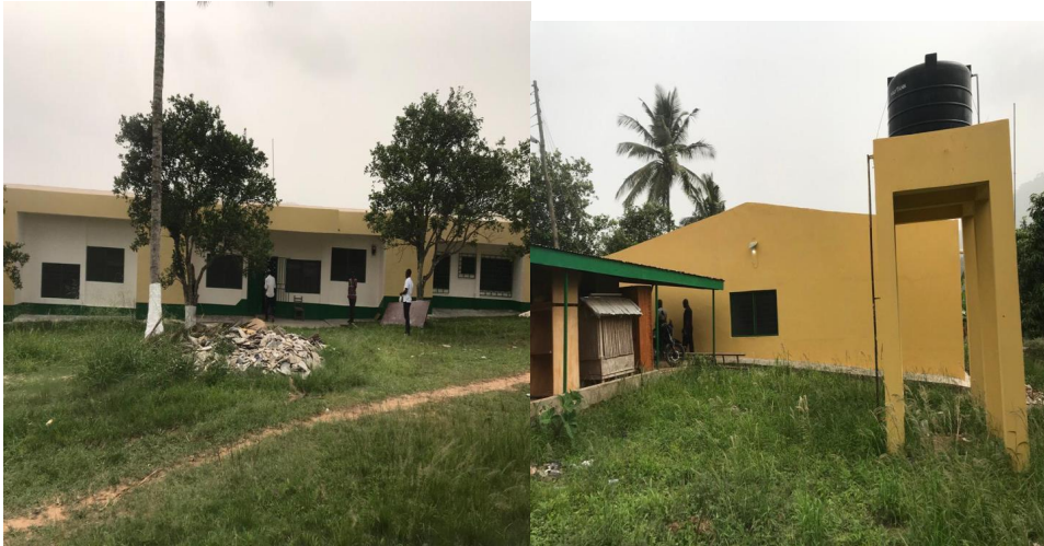
Renovation of Municipal Agric Office
