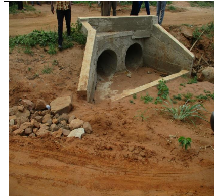
Completed 4No. 900 mm Culverts with approach filling at Hyewohoden
