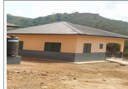
Completed 1No. CHPS Compound at Oframase
