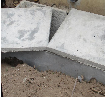
Completed 56No. Household Toilets with Bio Digesters at Asouyaa
