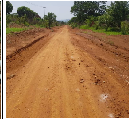
Reshaped 20km feeder road at Hyewohoden, Nkwakwasem and Bukuruwaa
