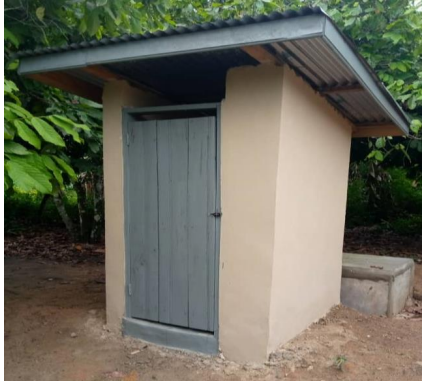
Completed 56No. Household Toilets with Bio Digesters at Asouyaa
