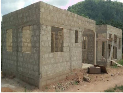
Completion of 1No. CHPS Compound with Out-House at Abisu. 55% Complete
