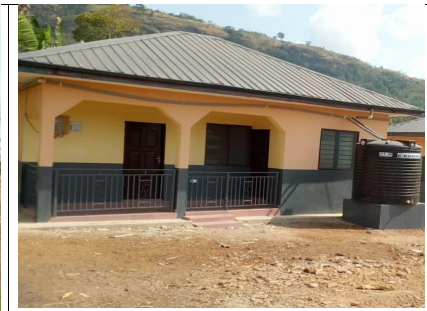
Completed 1No. Outhouse for CHPS Compound at Oframase.
