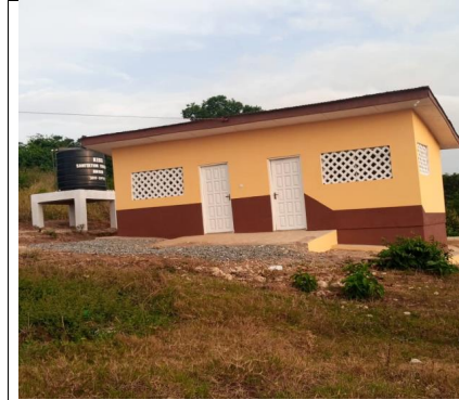
Completed 6-Seater W/C Toilet, Water System and Bio Digester at Abetifi Ridge School
