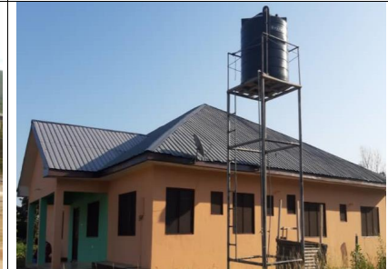
Completed 1No Imaging Center at Bokuruwa.
