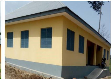
Completed 1No. CHPS Compound at Miaso
