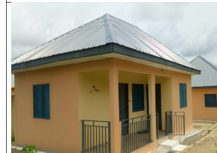
Completed 1No. CHPS Compound with Out-House at Mota
