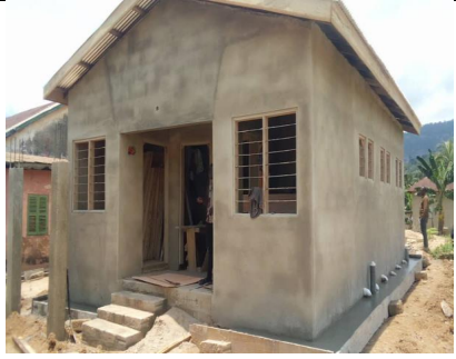
Construction of 12-Seater W/C Toilet with Water System at Akwasiho. 80% Complete
