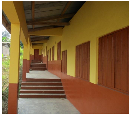
Completed 1No. 3-Unit Classroom Block, Urinal, KVIP and Office at Nkwatia.
