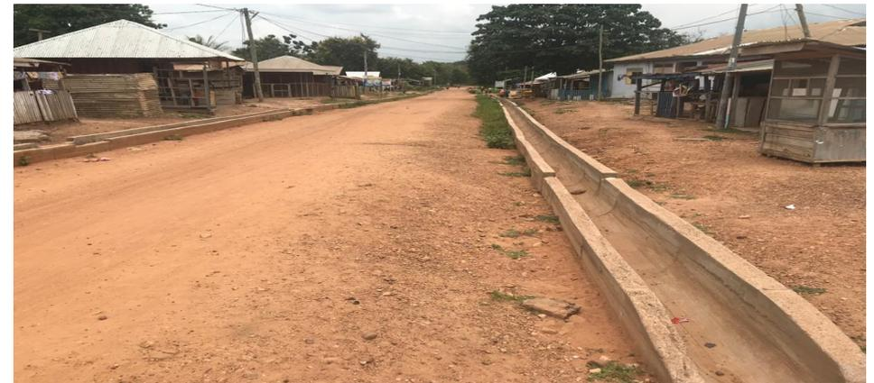
**Fig.5: 1230meter U-drain Constructed at Asikasu (75% Complete as at July 2021)**
