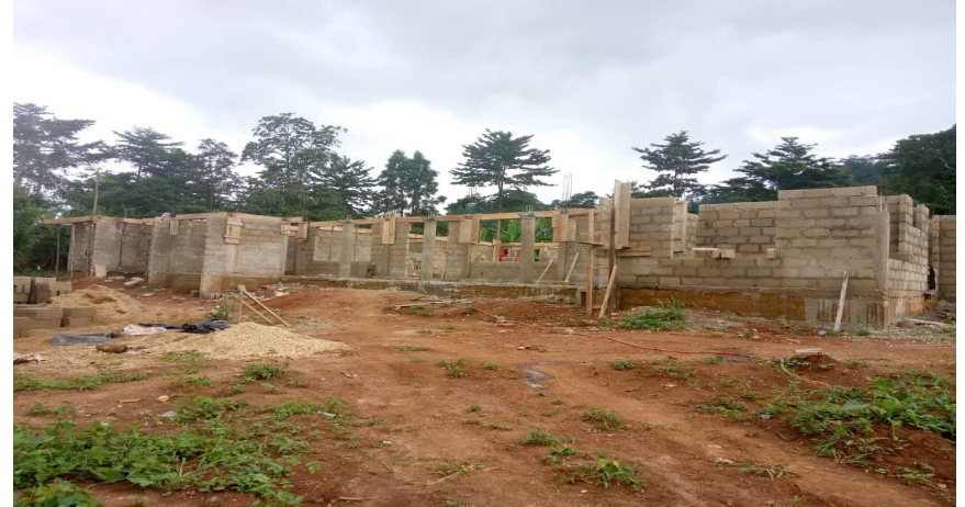
Construction of Magistrate Court at Akyem Osino (Funded By: MLGRD) – 60% Complete
