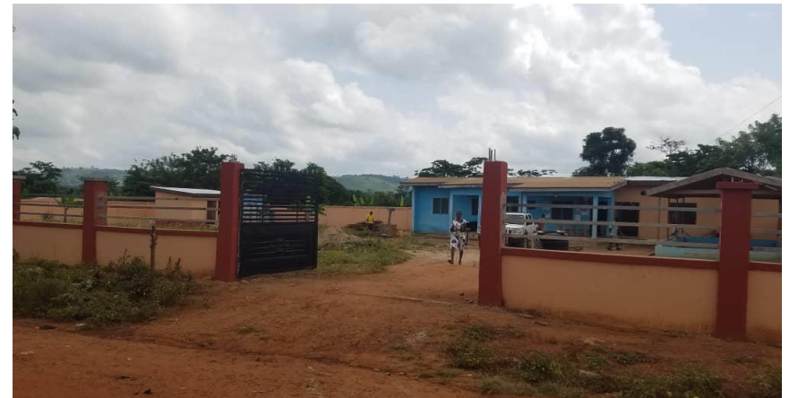
Renovated and fencing of Nkankama CHPS Compound (Funded By: World Vision)
