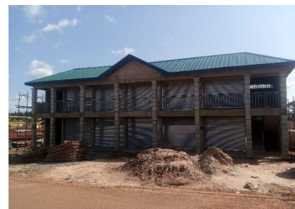
Construction of lockable stores at Aduasa
