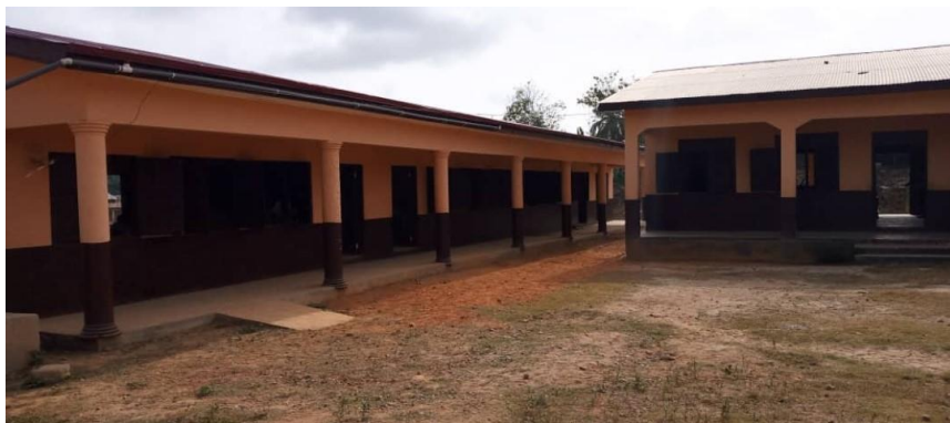
Completed School at Adiembra
