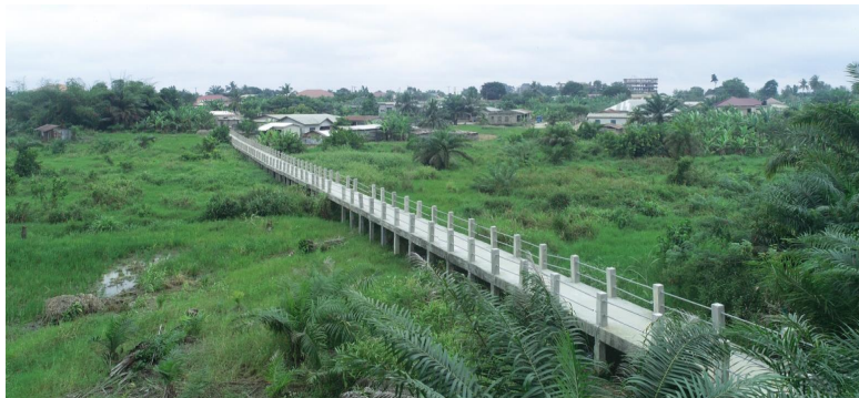
1NO FOOT BRIDGE CONSTRUCTED AT JESUS JESUS, AKIM ODA
