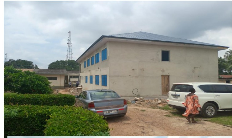
11NO. 2-STOREY MEDICAL LABORATORY ROOFED AND PLASTERED AT ODA GOV'T
