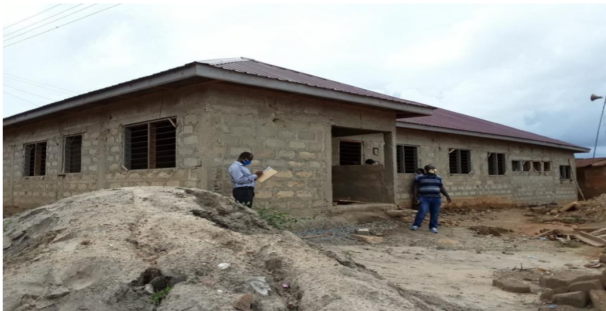
1NO. HEALTH CENTRE ROOFED AT ODA NKWANTA, - DACF
