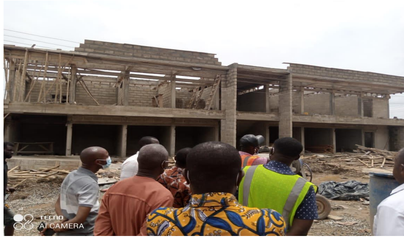
3NO. 34 NO. LOCKABLE MARKET STORES CONSTRUCTED TO GABLE STAGE AT NKWANTANUM, AKIM ODA - GSCSP
