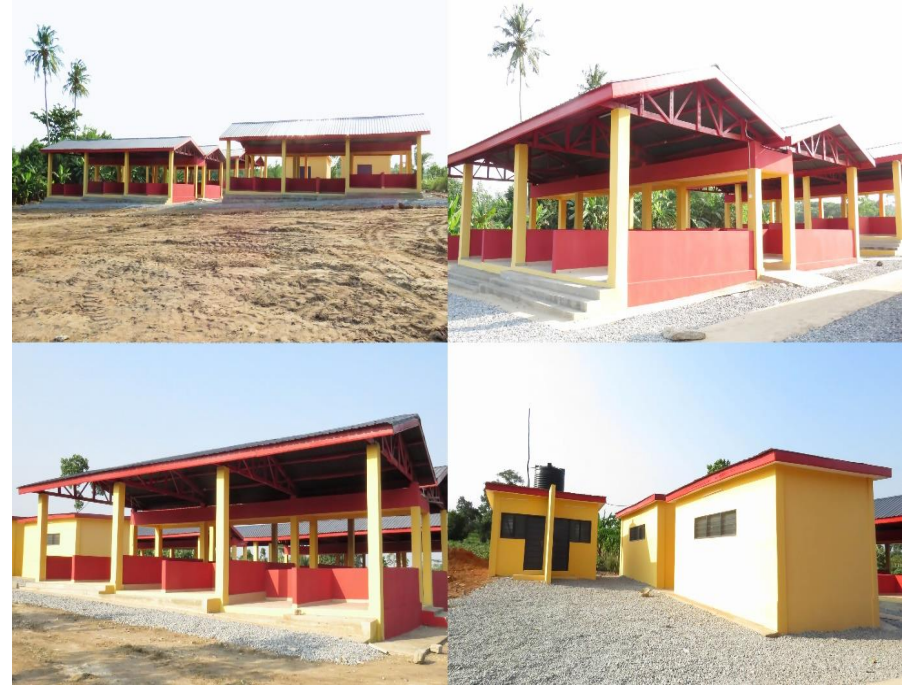
Constructed a Market Center at Kpakpotse
