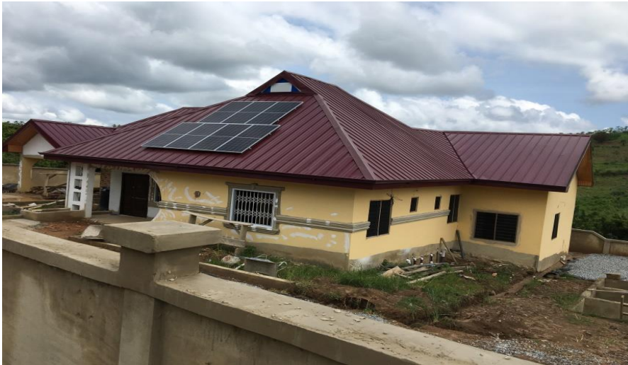
Constructed 1No. Judicial Service Bungalow for Ayensuano District Assembly at Coalta.
