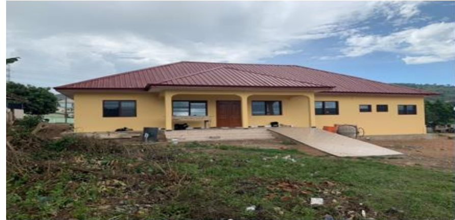
CONSTRUCTION OF CHPs COMPOUND WITH 2 NO. SELF-CONTAIN AT AKRADE
