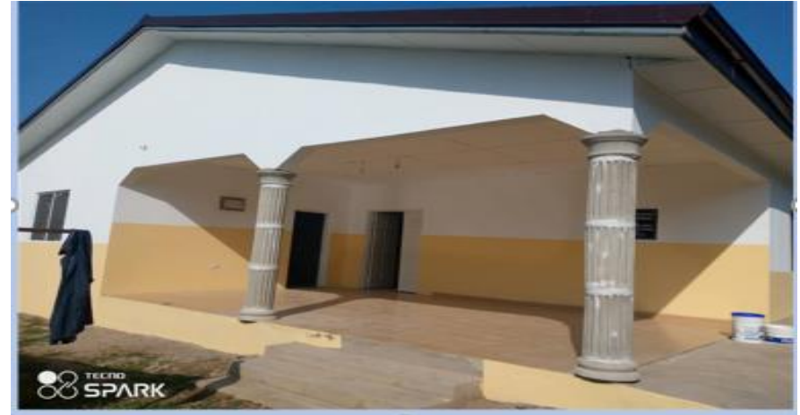
CONSTRUCTION OF 1 NO.8UNITS HOSPITAL WARD WITH OFFICE AT ANUM
