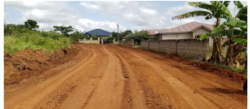
GRADING / GRAVELLING AND RESHAPING OF SELECTED ROADS AT OKORASE – ASOMDWE JUNCTION 1-10
