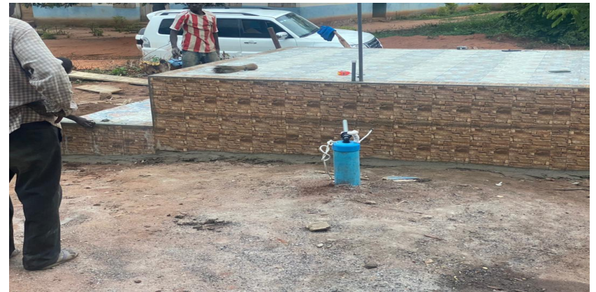
CONSTRUCTION OF A MECHANIZED BOREHOLE WITH RESERVOIR AT OBOM
