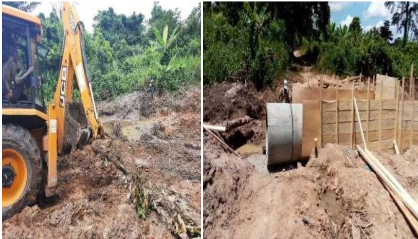
CONSTRUCTION OF A CULVERT ON ASUBOA RIVER (70% COMPLETE) – IGF
