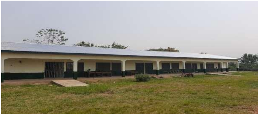
CONSTRUCTED 1No. 2-UNIT KG FOR ISLAMIC PRIMARY SCHOOL AT NEW TAFO
