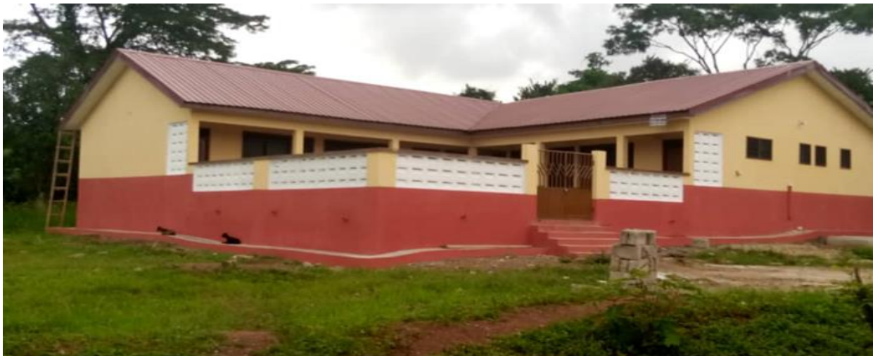
2-Unit KG block with office, kitchen and playing ground at Nkronua
