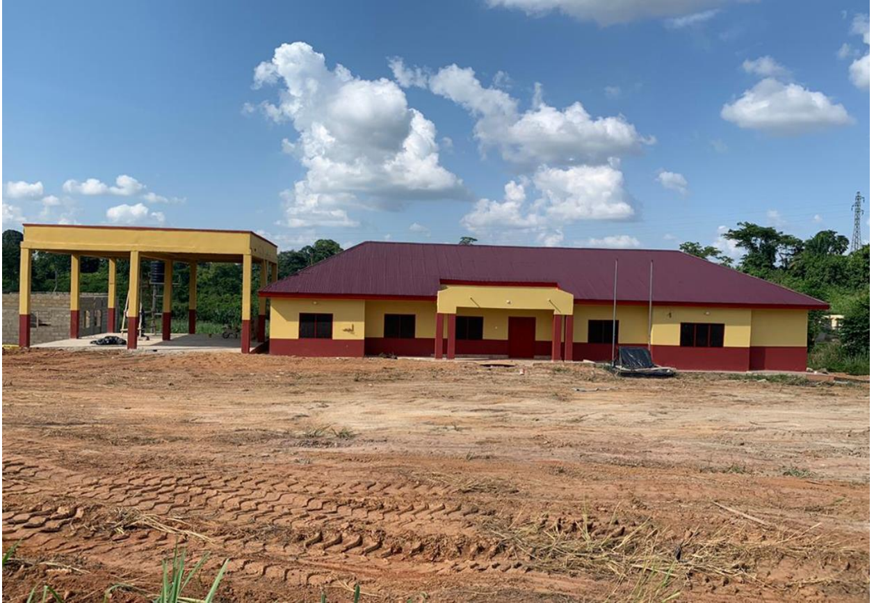
Fire and Ambulance Service Station at Diaso
