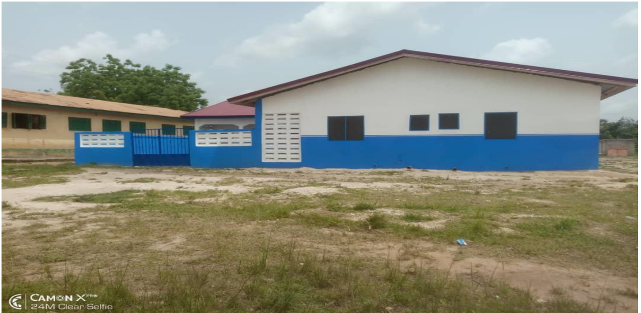
2-Unit KG block with office, kitchen and playing ground at Diaso Methodist school
