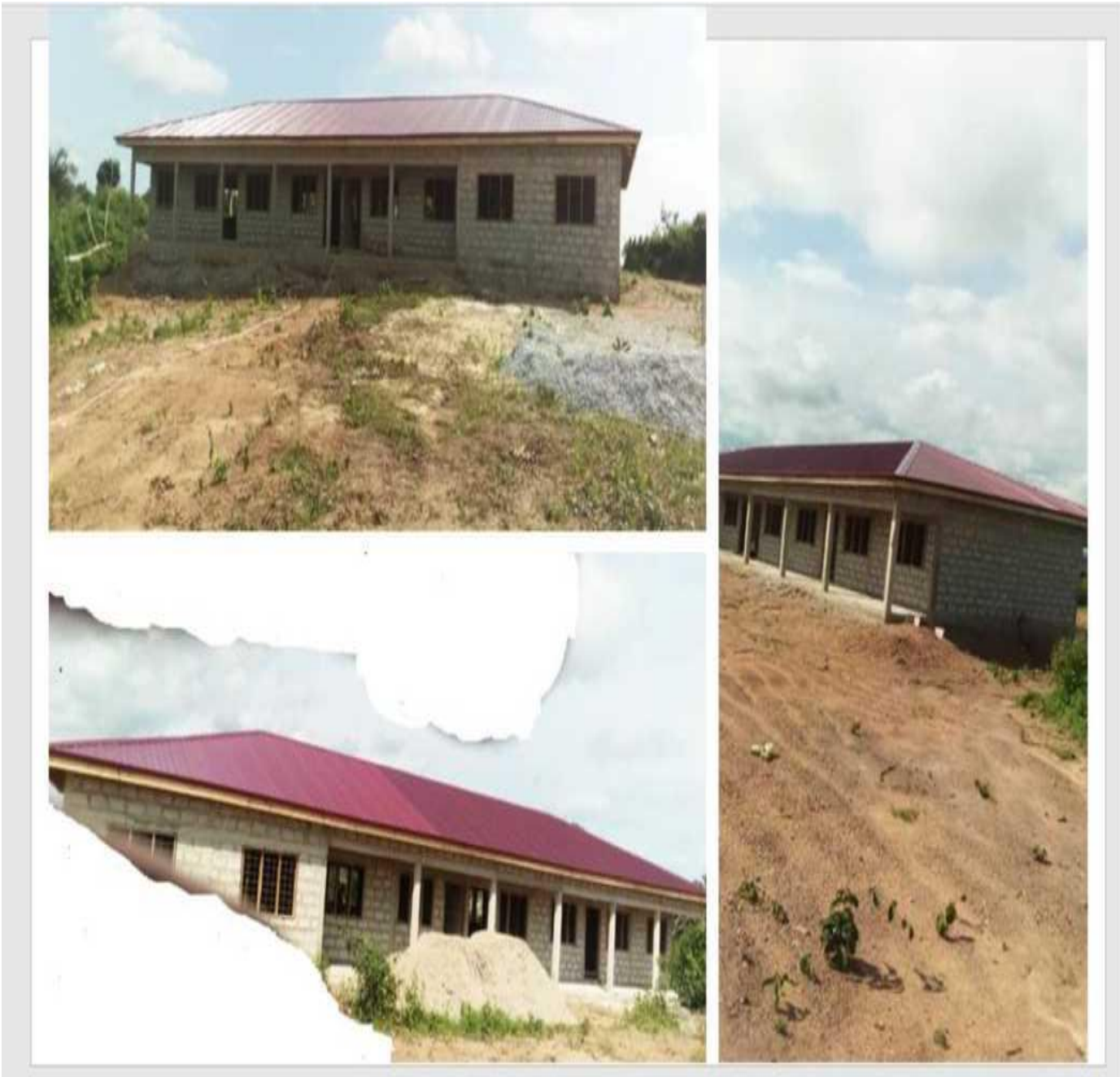
1No. 3Unit Classroom Block at Brabedze- 88% Completed (DACF-RFG)
