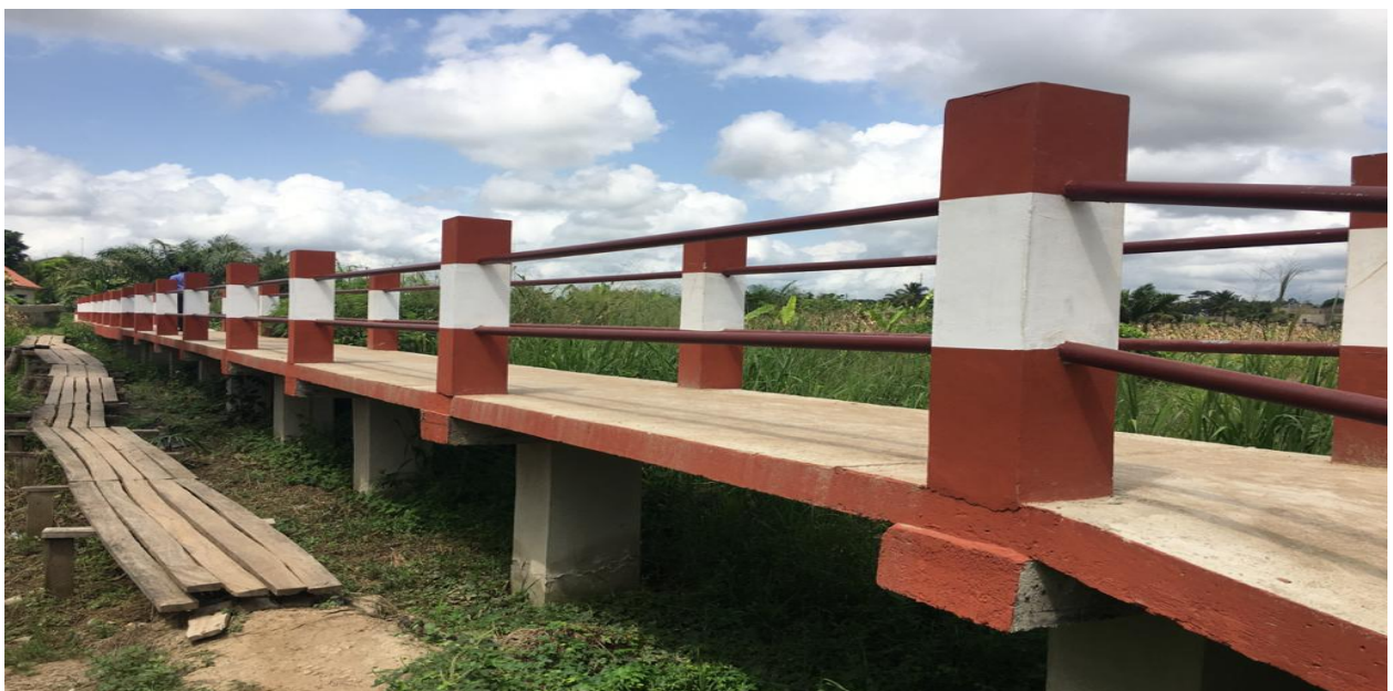
Figure 4: Constructed Footbridge and Dredged Ponpong River
