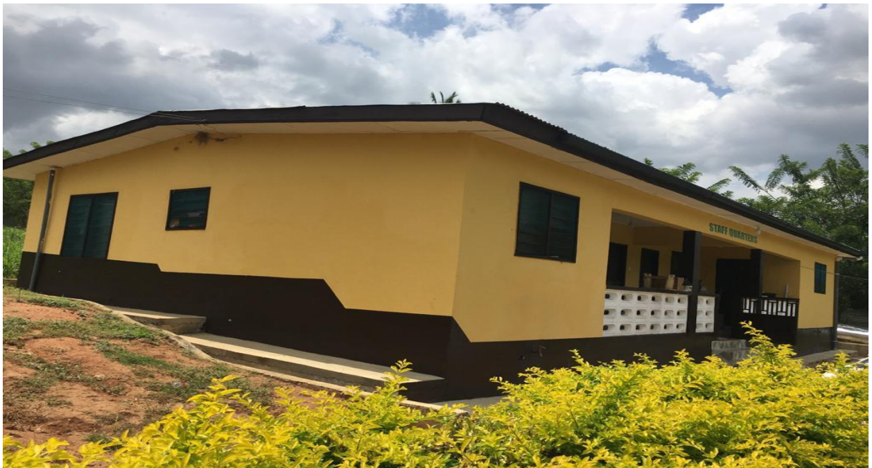
Figure 3: Rehabilitated Nurses Quarters at Bontrase Health Centre
