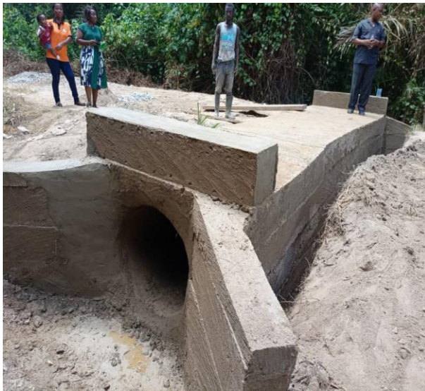
Const. of Pipe Culvert at Endwa-Dwenakyi
