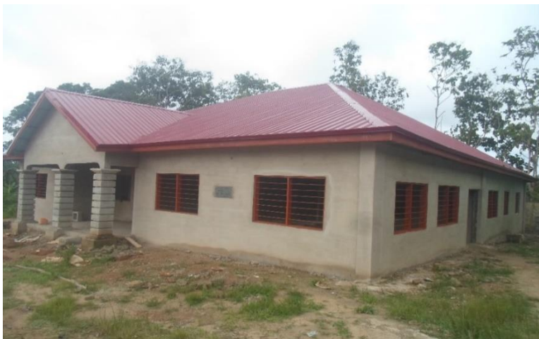
Construction of GES Annex at Breman Breman Asikuma
