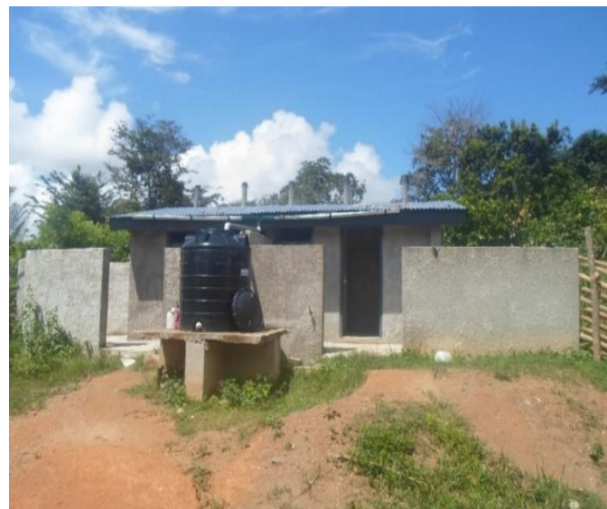
Construction of KVIP toilet at Ochisoa D/A School with auxiliary facilities at Ohyianhyeda
