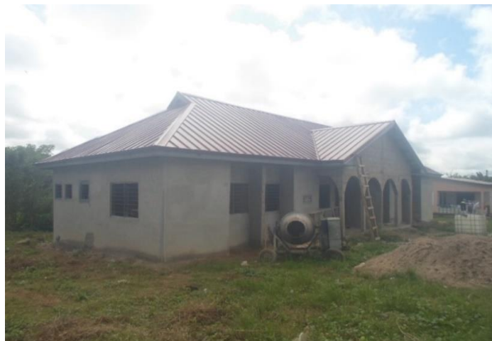
Construction of Nurses Quarters at Kojomensakrom
