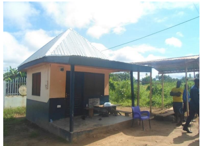
Construction of Police Post at Baako Road with IGF
