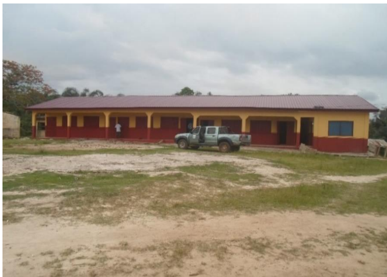
Construction of 1 No. 3 Unit Classroom Block
