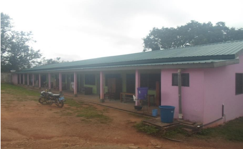
Renovation of PWD Office at Breman Asikuma
