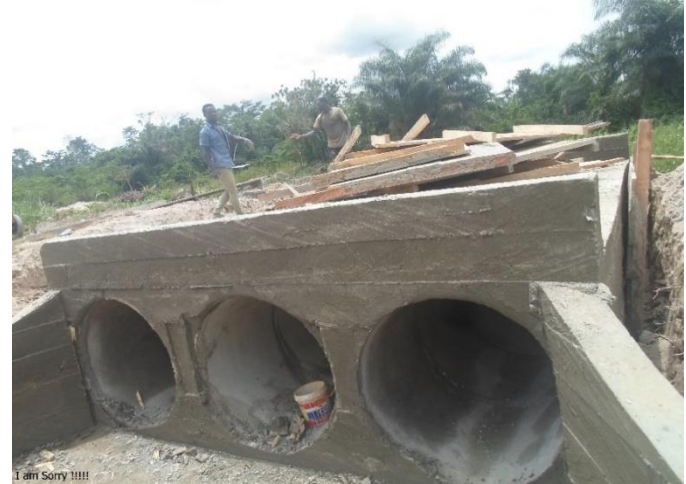
Construction of 1 No. Culvert at Adeambra
