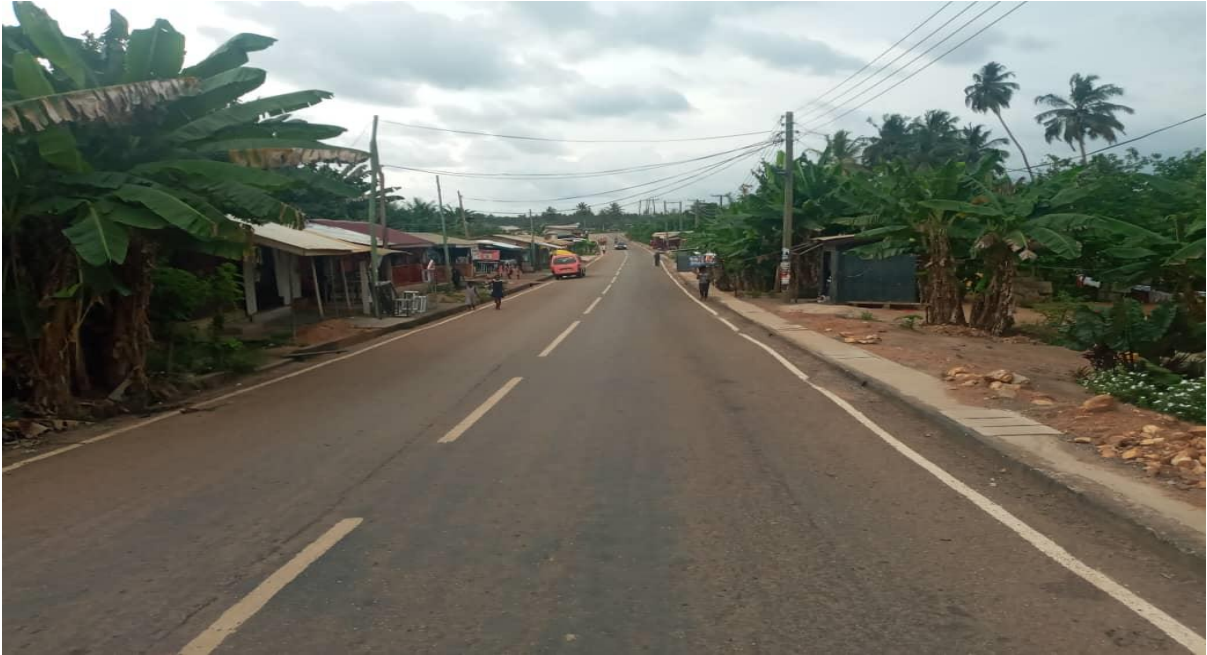
Bitumen surfacing on Esukontsen street (0.73km) Bitumen surfacing of
