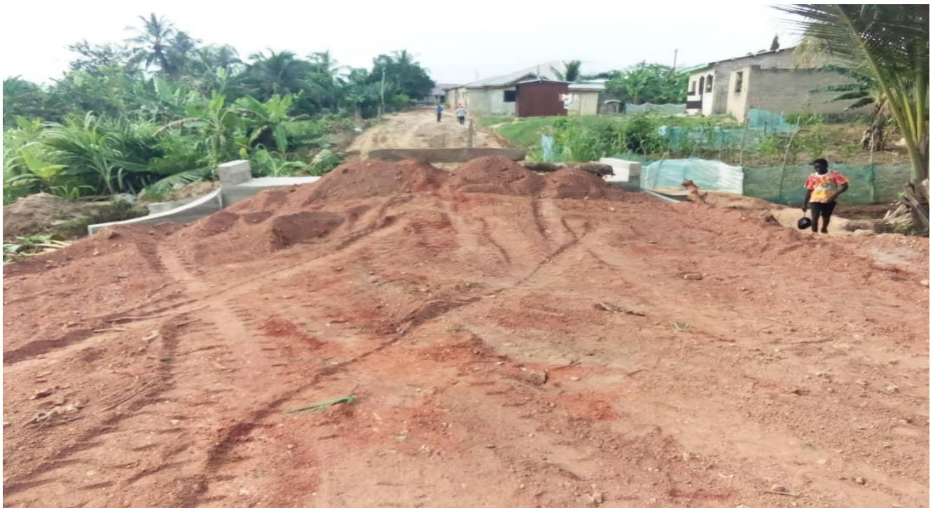
Culvert construction at Wawase
