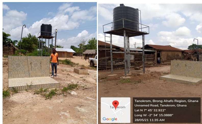
10 no Boreholes Drilled and Mechanised—DACF-RFG
