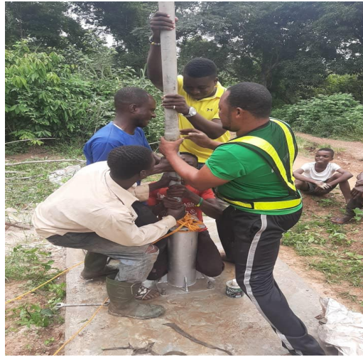
DRILLING AND INSTALLATION OF 4NO. HAND PUMPS AT AKURAKESSE, WHO KNOWS, AZUMAKROM AND APESIKA NO.1
