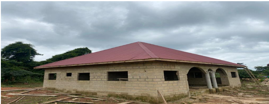
CONSTRUCTION OF 1NO. CHPS COMPOUND AT APRAKUKROM
