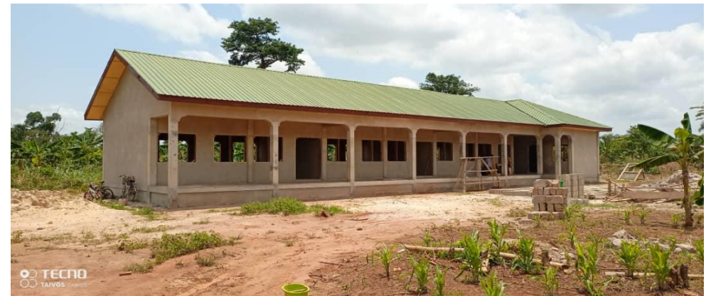
3Unit Classroom Block Constructed at Yawusukrom (75%)
