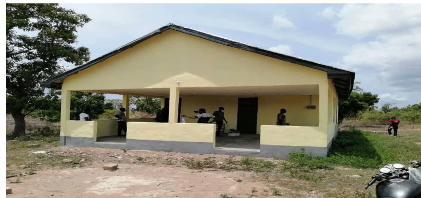
Constructed CHPS Compound at Gbli Wanzam
