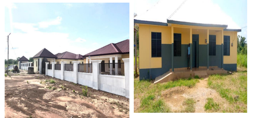
REGIONAL FEEDER ROADS STAFF QUARTERS-GOG CHPS COMPOUND AT BRONIKROM-DACF-RFG
