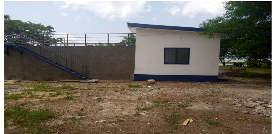
Rehabilitated Yeji Water System (CWSA)
