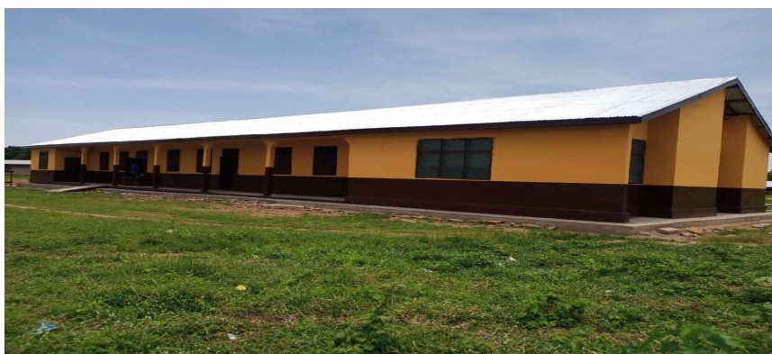
Rehabilitated 1No. 3unit classroom block at Konkoma (DACF)
