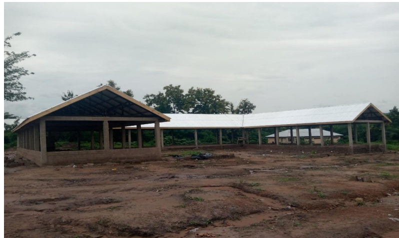
CONSTRUCTION OF 1N0. COMMUNITY SOCIAL CENTRE AT AMPOMA
