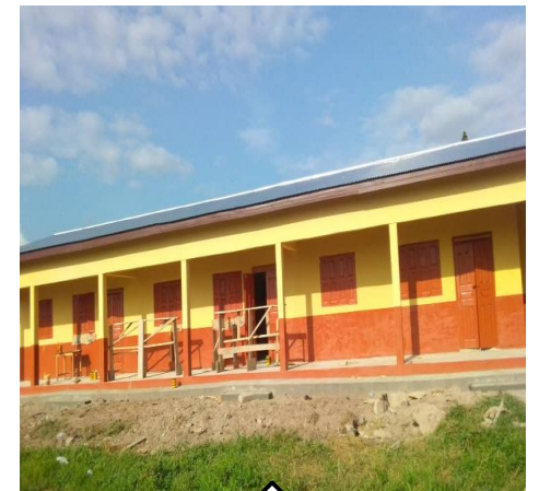
Completed and furnished 3-Unit Classroom Block with Auxiliary Facilities
