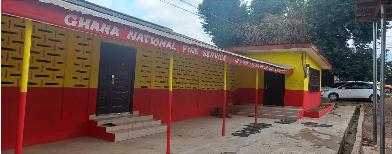
Construction of District Office for Fire Station and Ambulance Service at Agona
