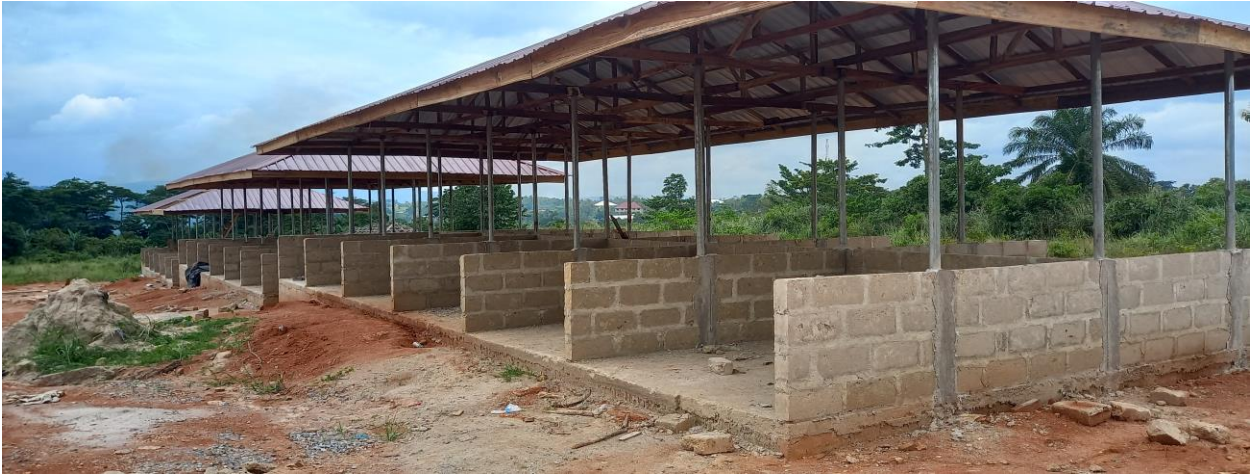
Construction of Lockable Market Stores At Agona
