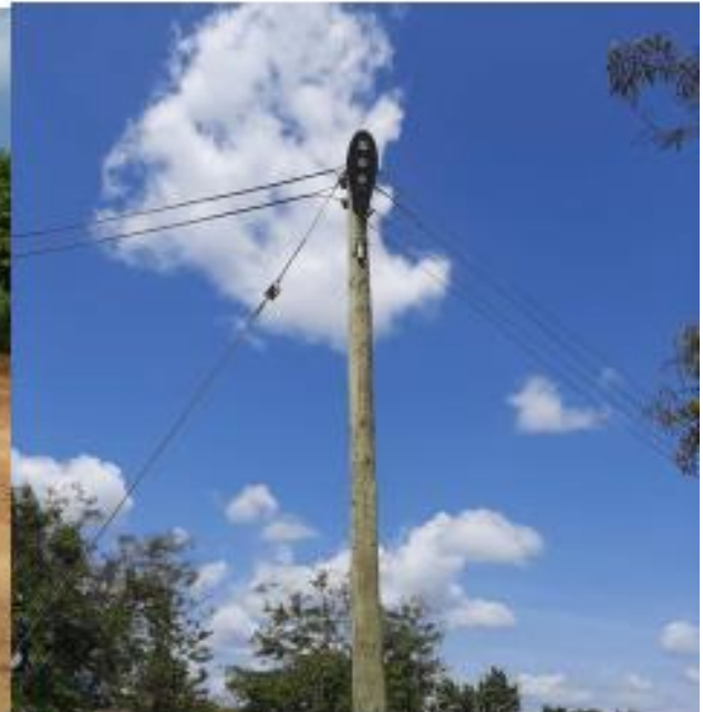
SUPPLIED AND INSTALLED 100NO. STREETLIGHTS DISTRICT WIDE
