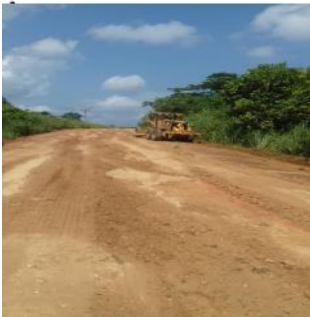
Reshaped 4km feeder roads – Senchi-Attakrom
