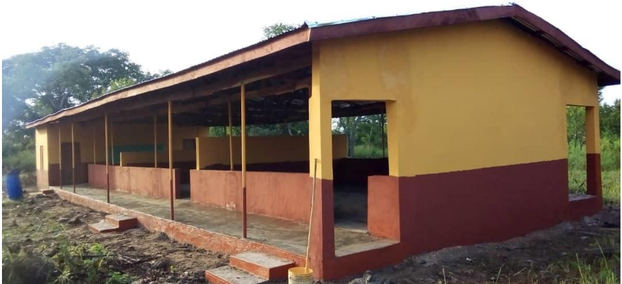
Constructed 1No 3-unit pavilion
