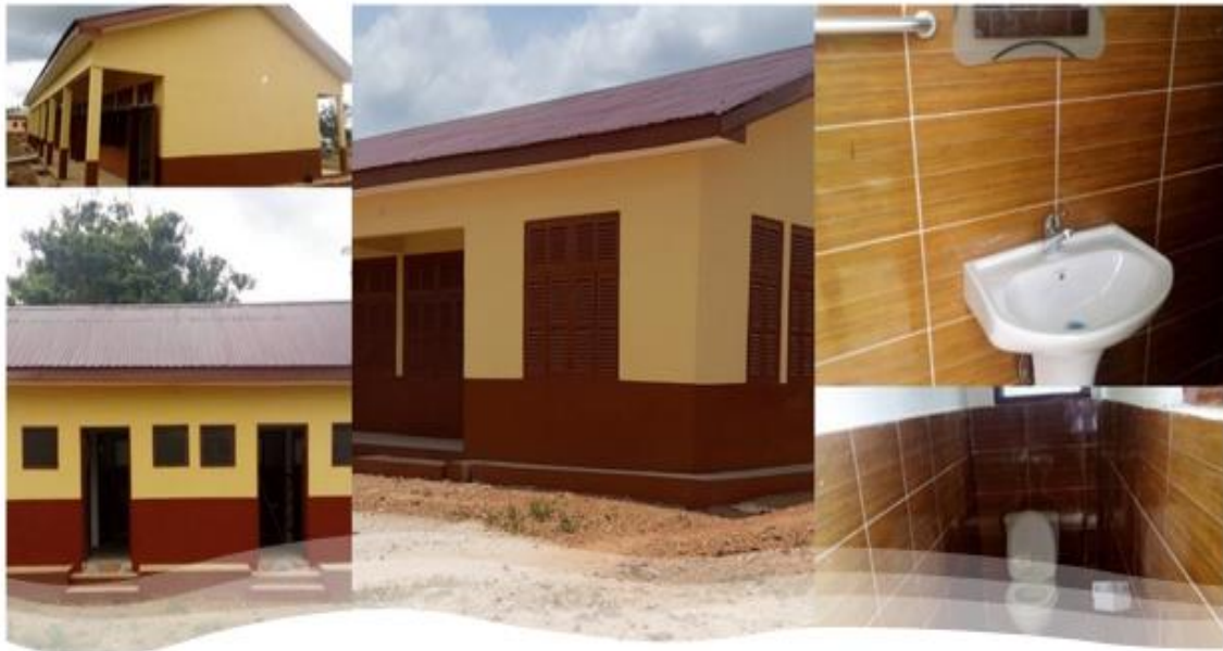
COMPLETED 3 UNIT CLASSROOM BLOCK WITH ANCILARY FACILITIES AT ADAASE
