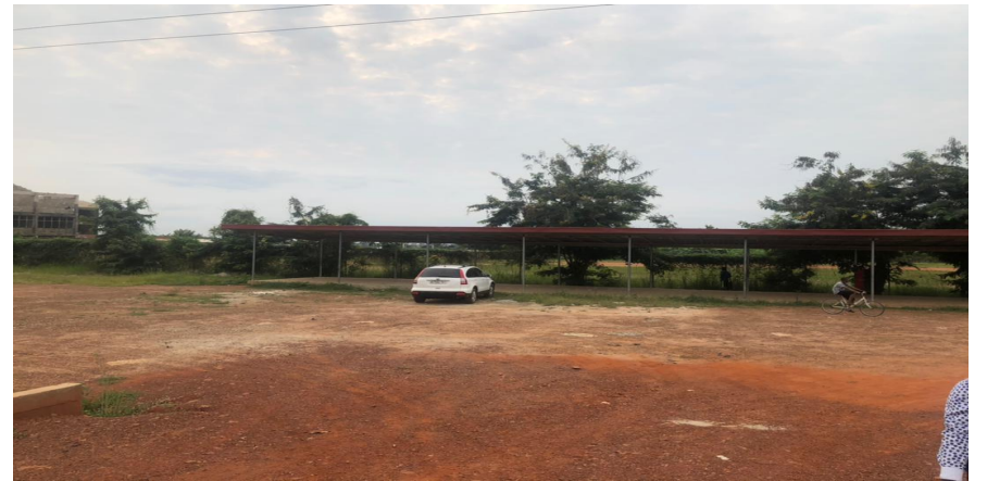
Construction of Lorry Park Terminal at Nkawie
