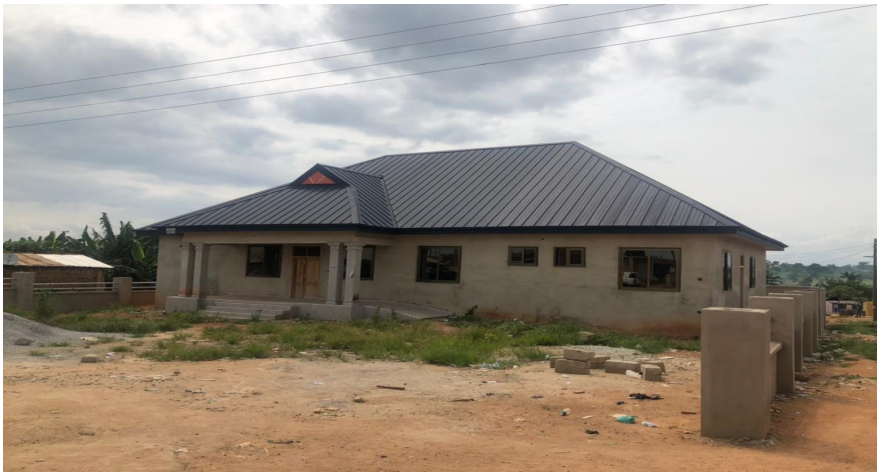
Construction of Police post at Sepaase
