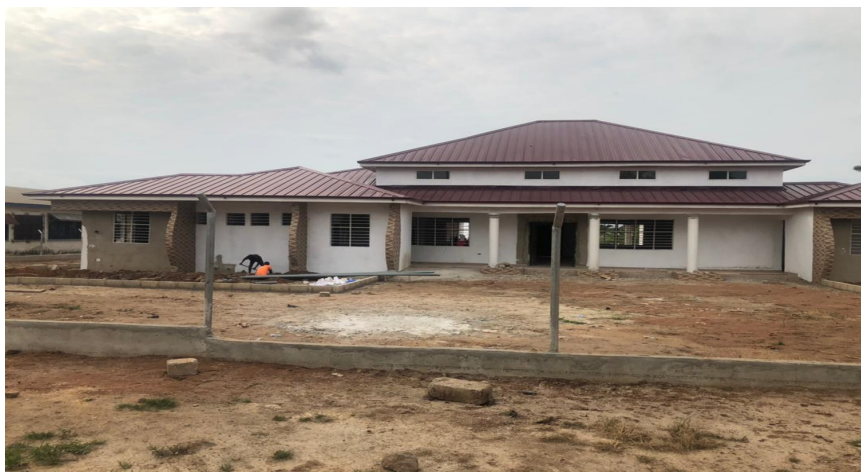
Construction of Court Building at Toase
