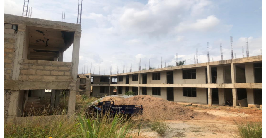
Construction of 18unit classroom block at Nkawie
