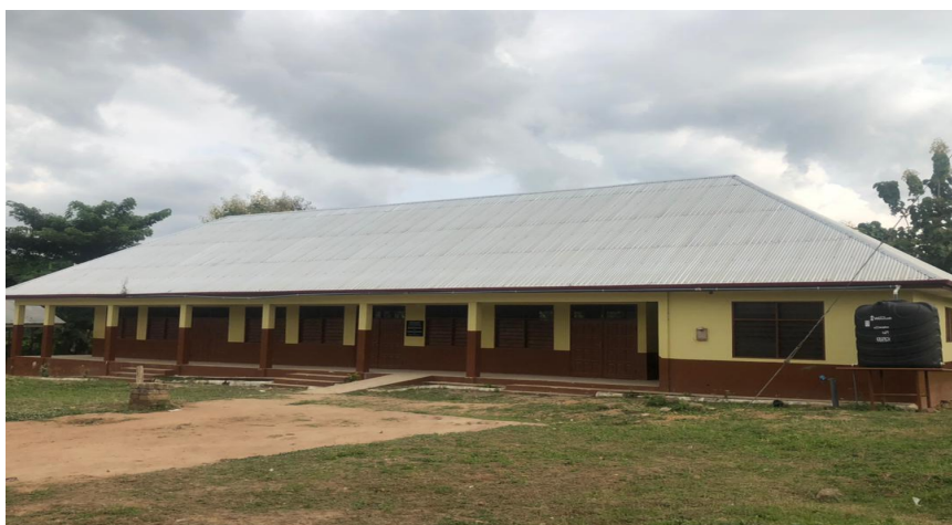
Construction of 1no. 3unit classroom block at Kyereyaase
