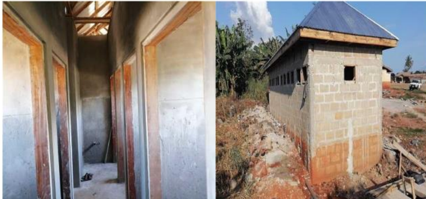
1. 1NO. 20 SEATER ACQUA PRIVY TOILET WITH MECHANIZED BOREHOLE AT KENTENKYIRE
