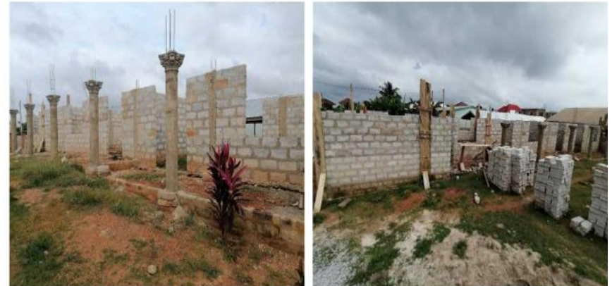
3. 1NO. 3UNITS CLASSROOM BLOCK AT AFASIEBON
