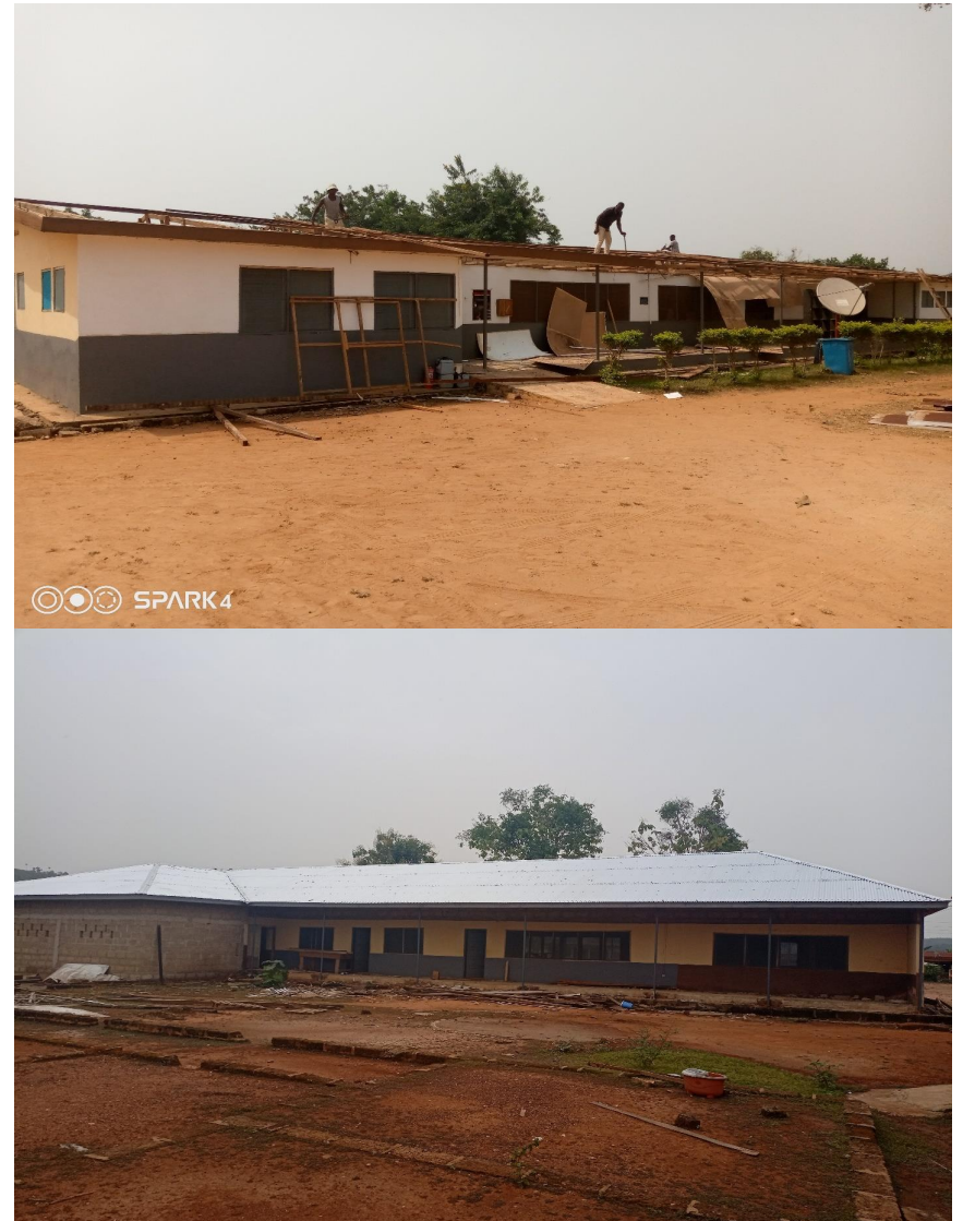
RENOVATION OF HEALTH CENTRE AT NYINAMPONASE
