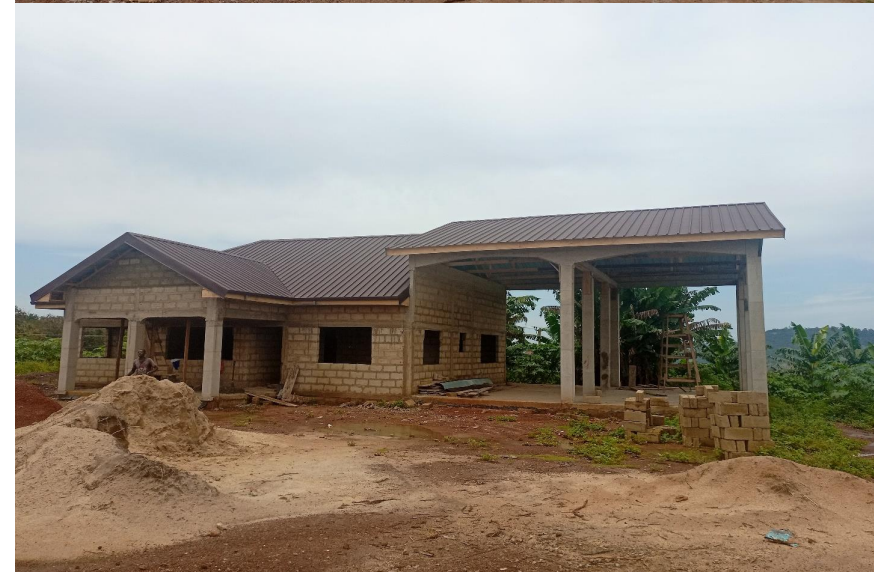
CONSTRUCTION OF FIRE STATION AT AGOGO
