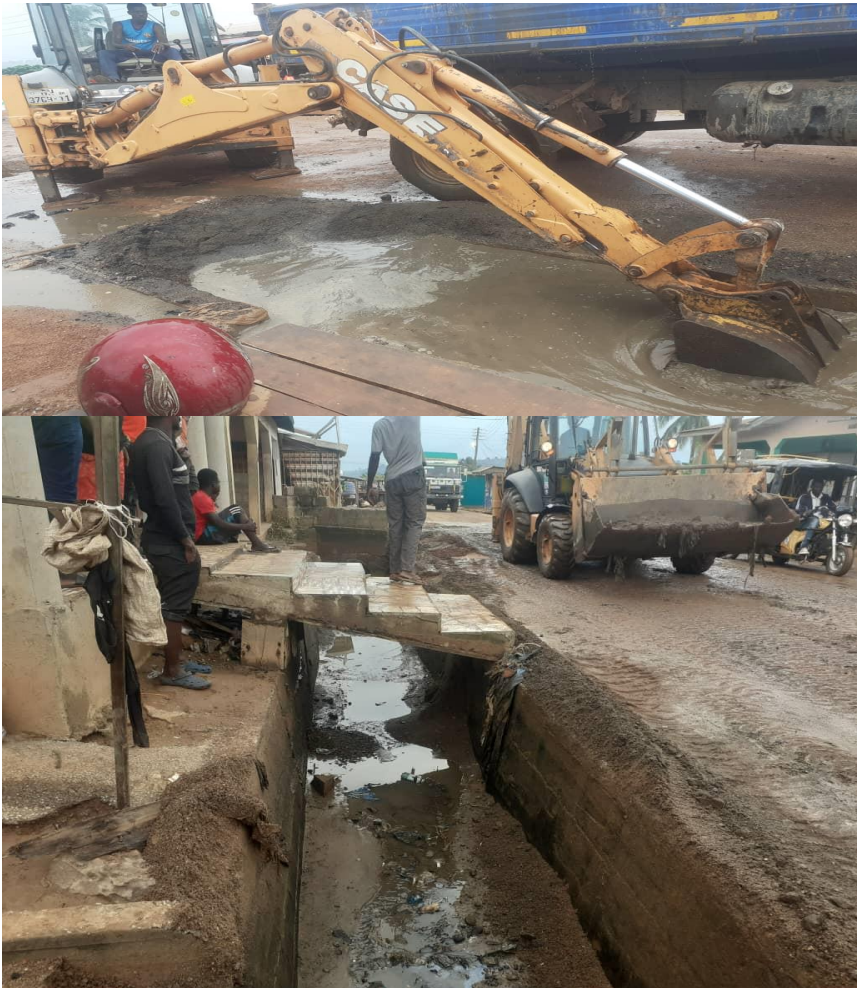
DISILTING OF DRAINS AT AGOGO
