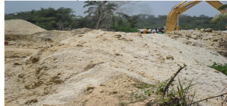
Plate 4: Sand Dumped for reclamation
