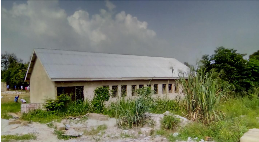
ADUMAN SHS WC
