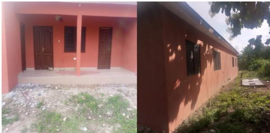
Construction of Teachers Quarters at Meduma (DACF-RFG)
