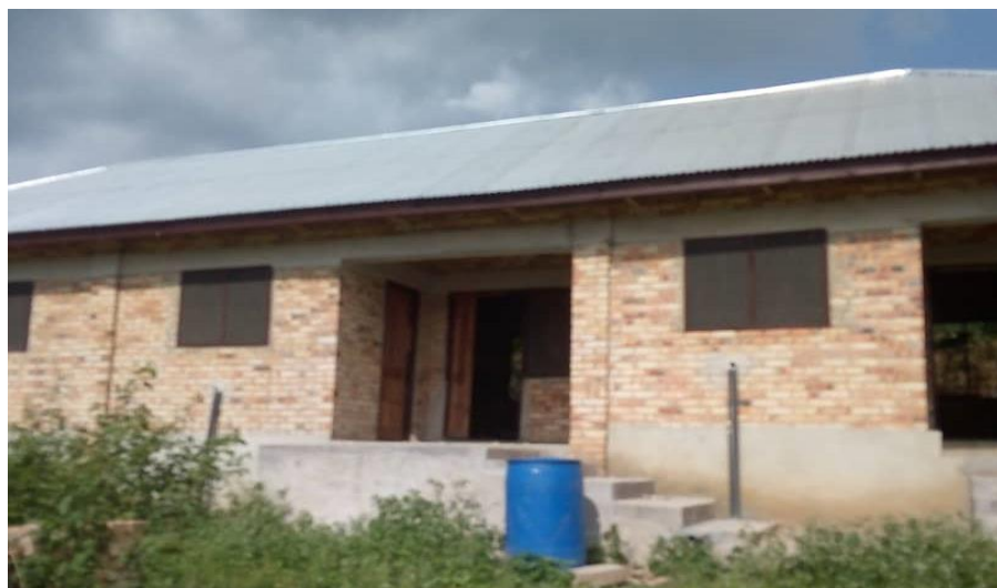
Constructed Teachers Quarters at Kusa
